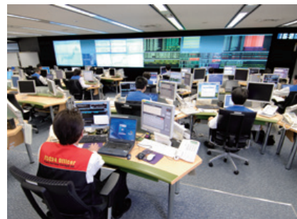
FSC24, a command-and-control center for monitoring, maintenance and operations
